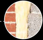
Increased Cavity Wall Thickness
